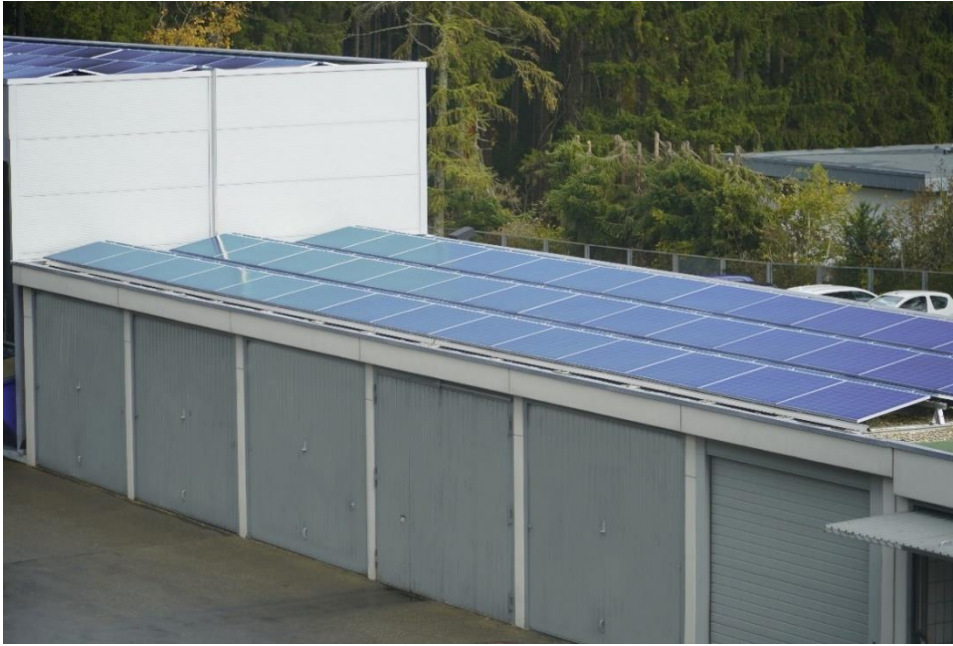
Installation of a PV system (garages and container storage area)
