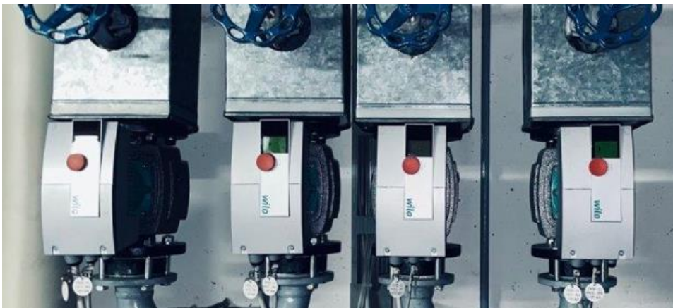
Conversion to regulated pumps
