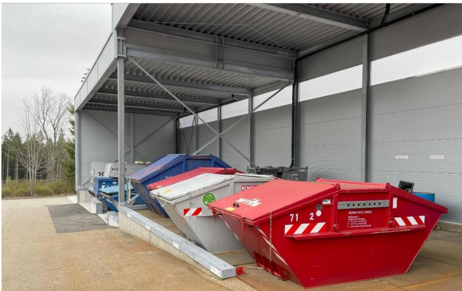
Roofing of the container storage area
